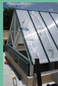
Skylights are nearing completion on medical and residential buildings.
