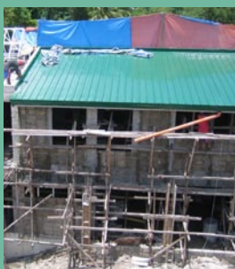
Right: Roofing is completed on both buildings
